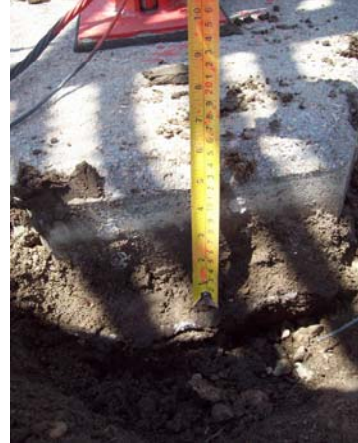
Determining dimensions of base spreadfooting by using probe
