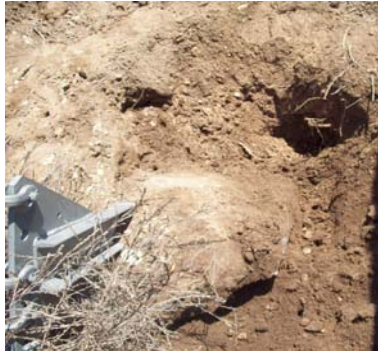
Concrete encasement around anchor rods
