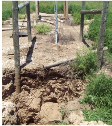
Anchor block exposure
